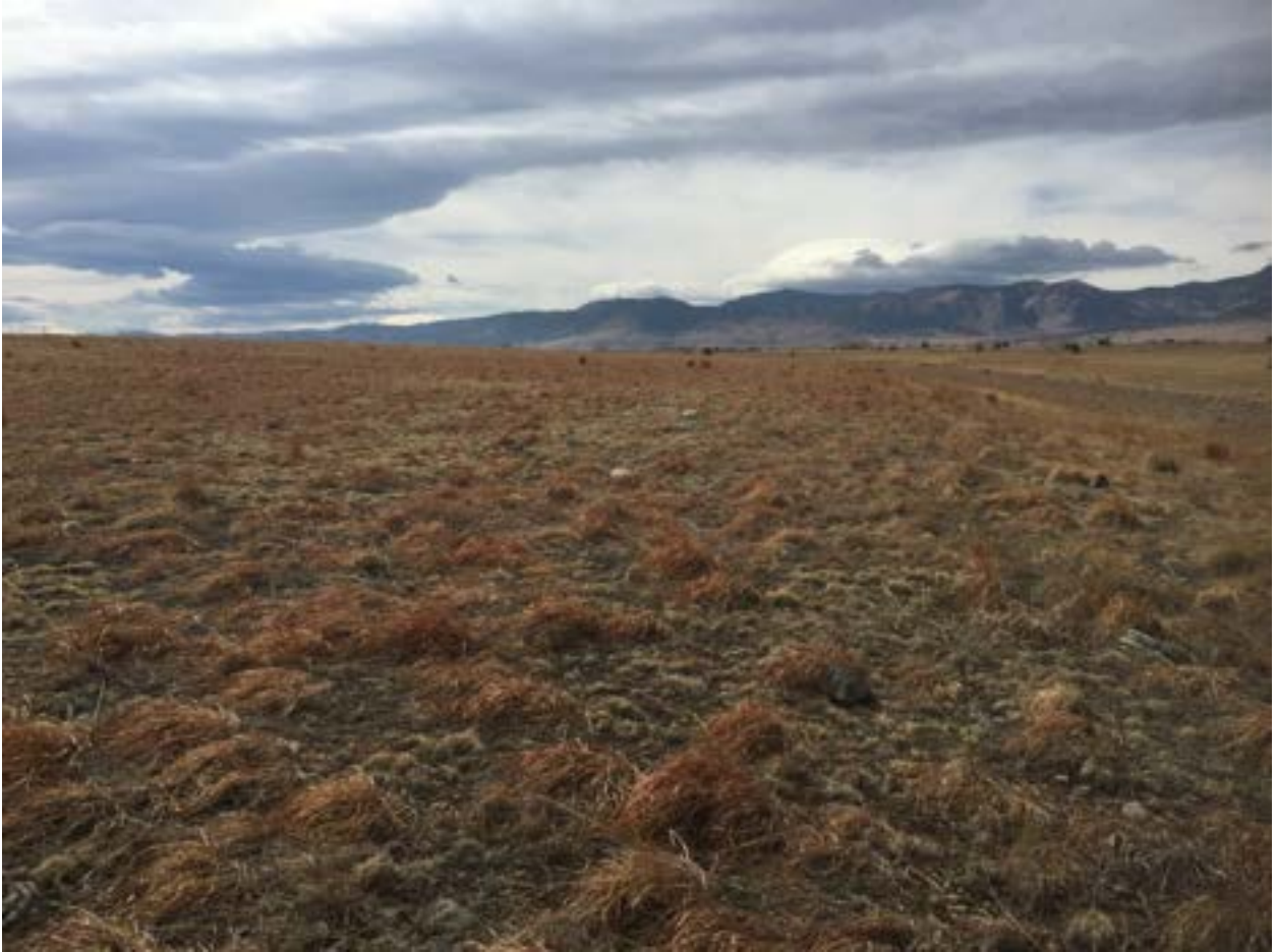
PLF Looking West at the Cover Side Slope – North
