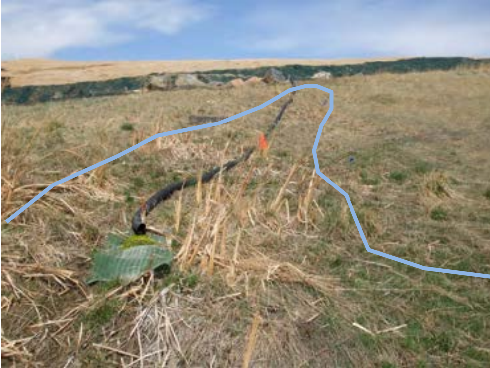
Figure 6. Standing Below the Seep 2/3 Drainage Outfall Looking North at the Wet Area Discovered (estimated outline in blue)
